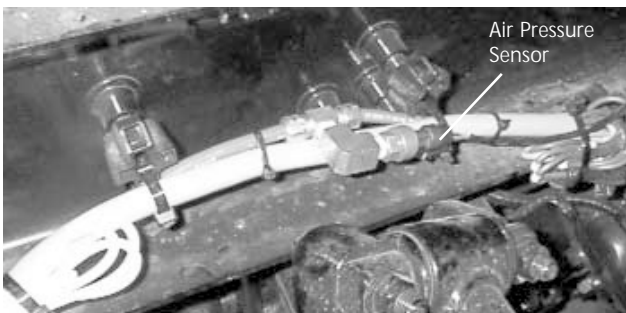
Fig. 6: Air Pressure Sensor Completed Installation
